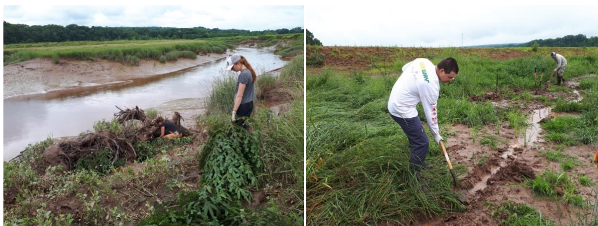
Figure 1.26 Adaptive management practices being undertaken at the Belcher St realignment site, 2019 (1.26a left: runnels being dug by hand; 1.26b right: living shoreline repair; TransCoastal Adaptations Centre for Nature-Based Solutions)
