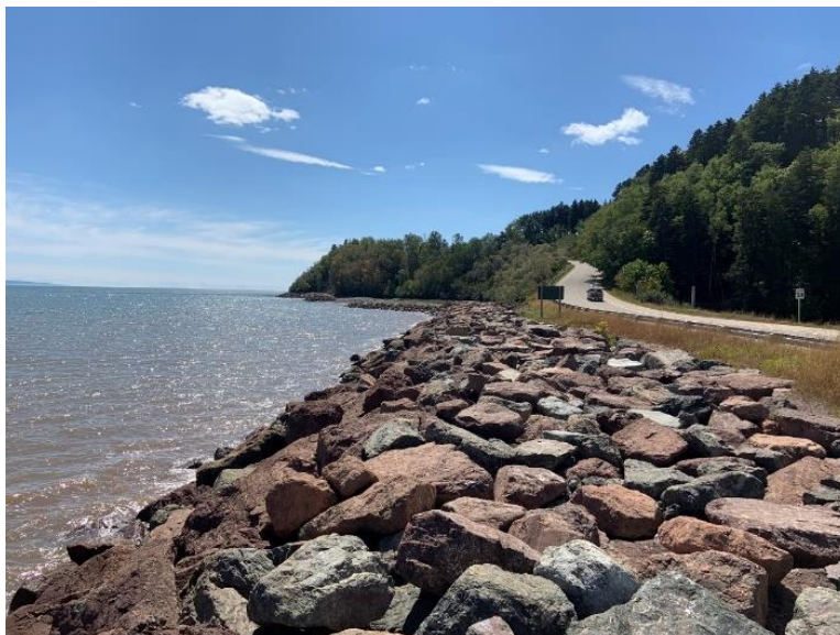
Figure 1.16 Armourstone Revetment in Fundy National Park, NB (Vincent Leys, CBCL Ltd.)
