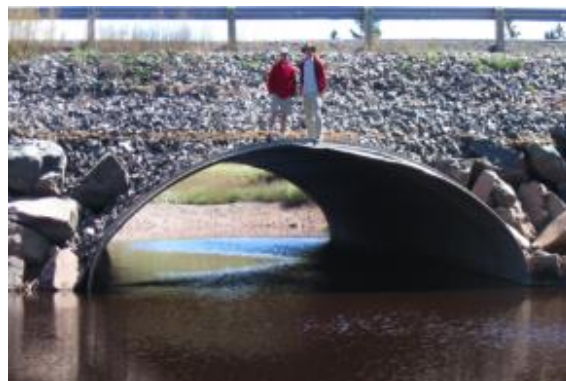
Figure 1.14 Cheverie Creek culvert pipe, Cheverie, NS (Tony Bowron, CBWES Inc.)
