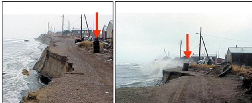
Figure 2.50 Example of how monitoring with images can inform decision-makers on coastal changes such as erosion. The above image was taken in Shishmaref, Alaska where melting permafrost has increased coastal erosion (T. Weyiouanna 283 )
