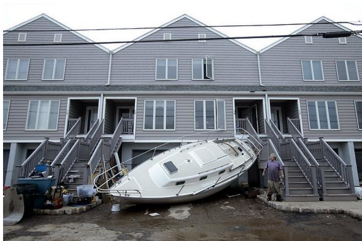
Figure 3.48 Impact on this flood-proofed housing is minimal despite major impacts on Sea Bright shoreline infrastructure as indicated by the beached sailboat
