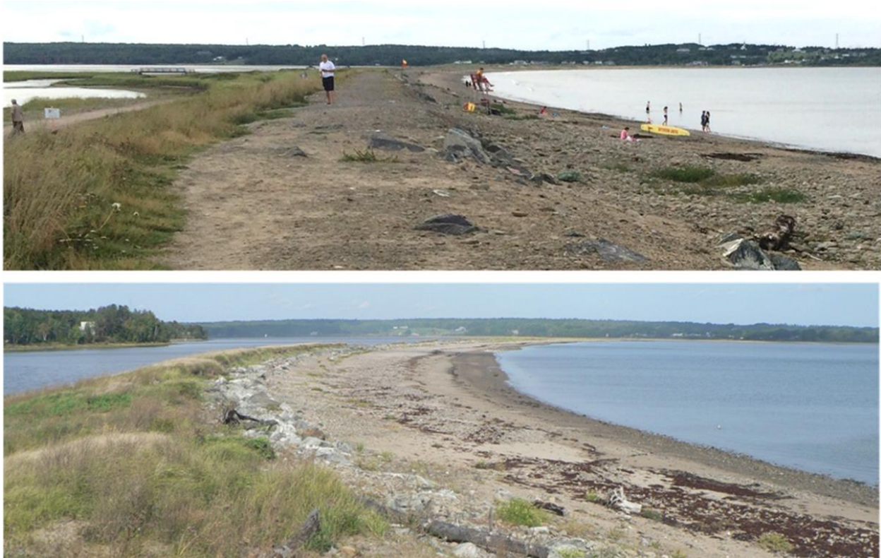
Figure 3.12 Buried revetment at Dominion Beach, NS, two years after construction (top), and Lighthouse Beach, NS, six years after construction (Vincent Leys, CBCL Limited)
