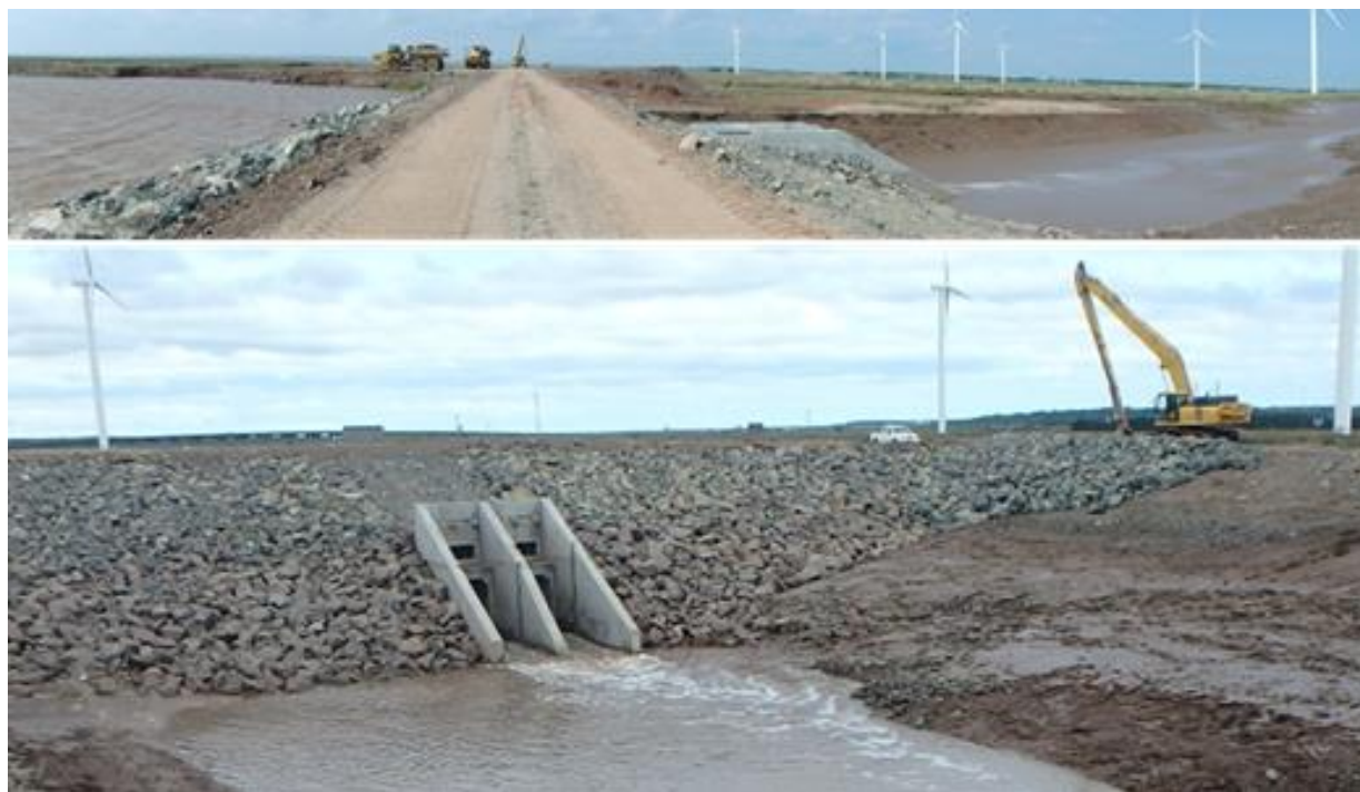
Figure 3.44 La Planche River Aboiteau near completion, August 2015 (Suvir Pursnani, CBCL Limited)
