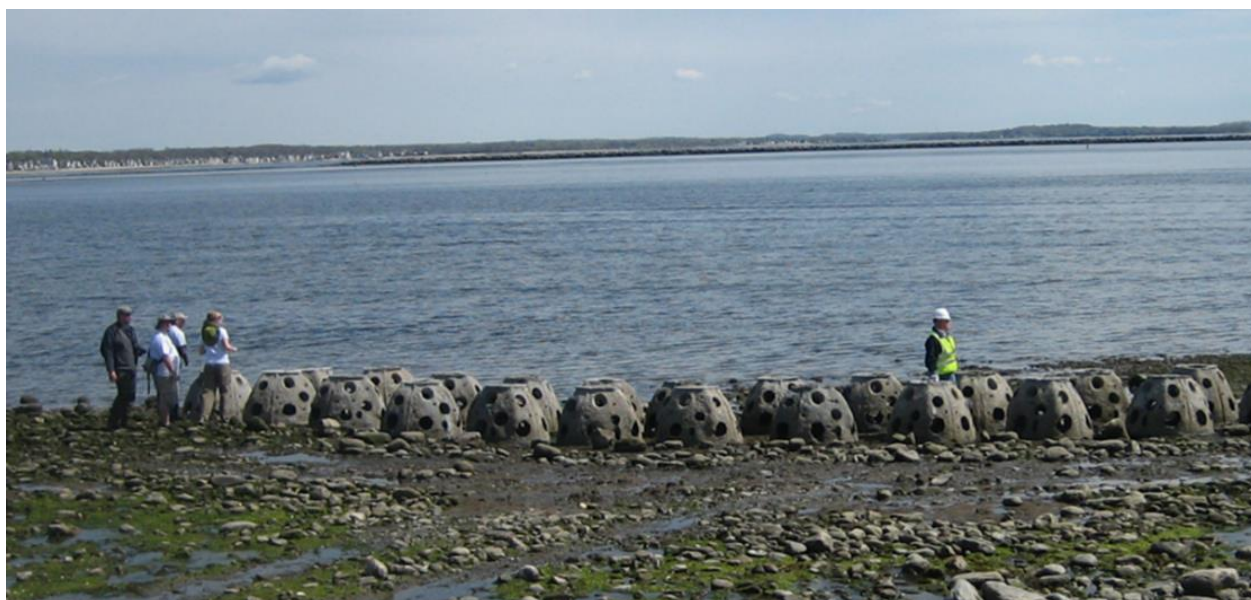
Figure 3.10 Concrete reef balls (Paul Stern, 2014)
