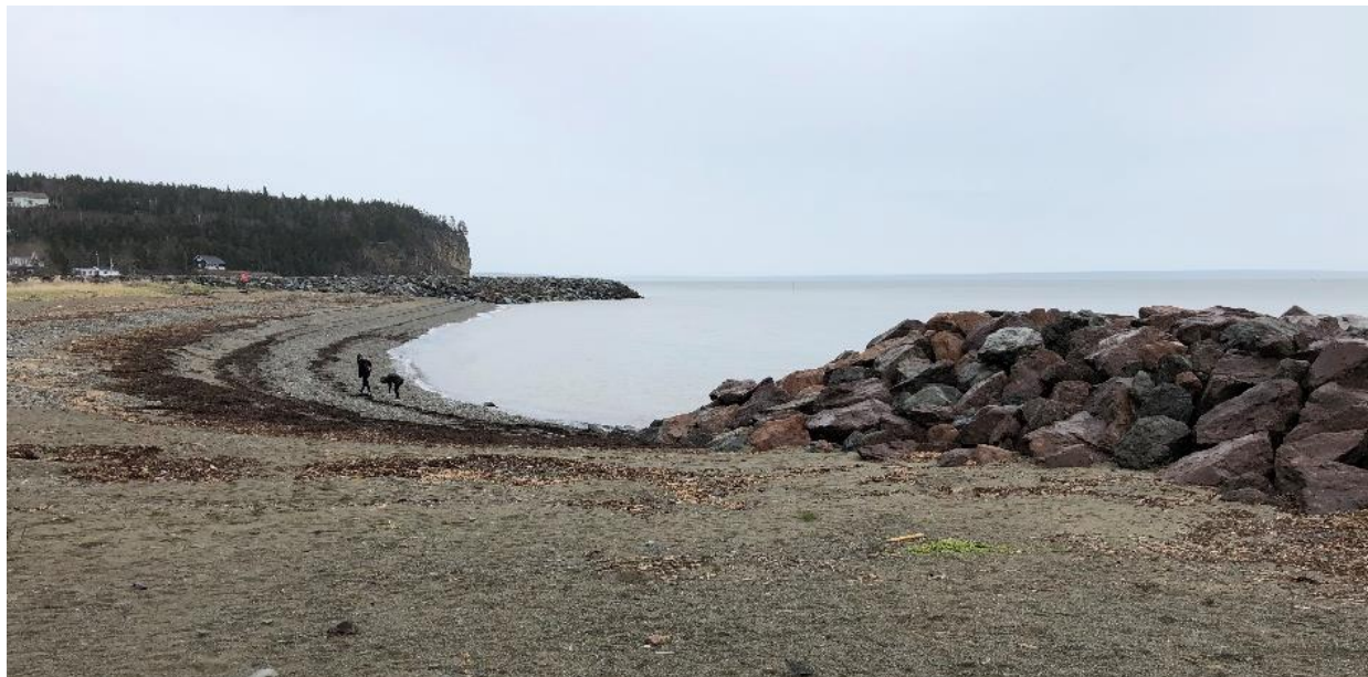
Figure 3.33 Breakwaters at Fundy National Park (Vincent Leys, CBCL Limited)
