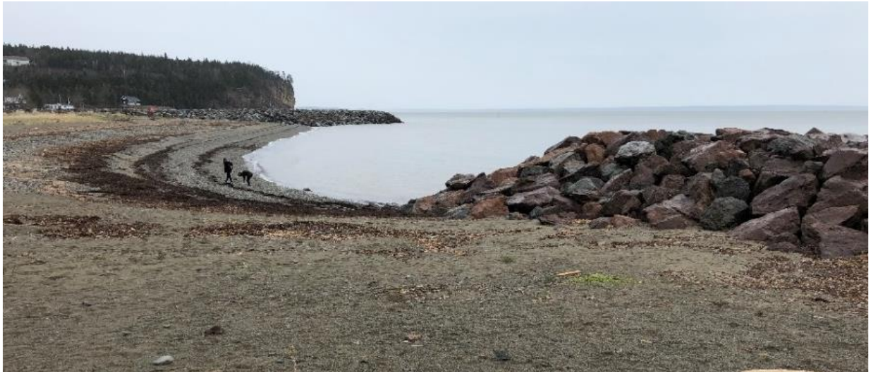
Figure 3.15 Beach stabilization breakwaters at Fundy National Park, NB (Vincent Leys, CBCL Limited)
