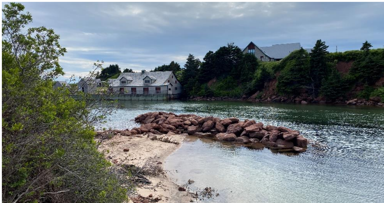
Figure 3.41 T-Head groyne at Basin Head Provincial Park, PEI (Vincent Leys, CBCL Limited)
