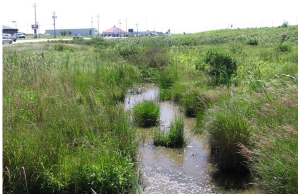
Figure 3.28 Grass swale in Yarmouth, NS (Alexander Wilson, CBCL Limited)
