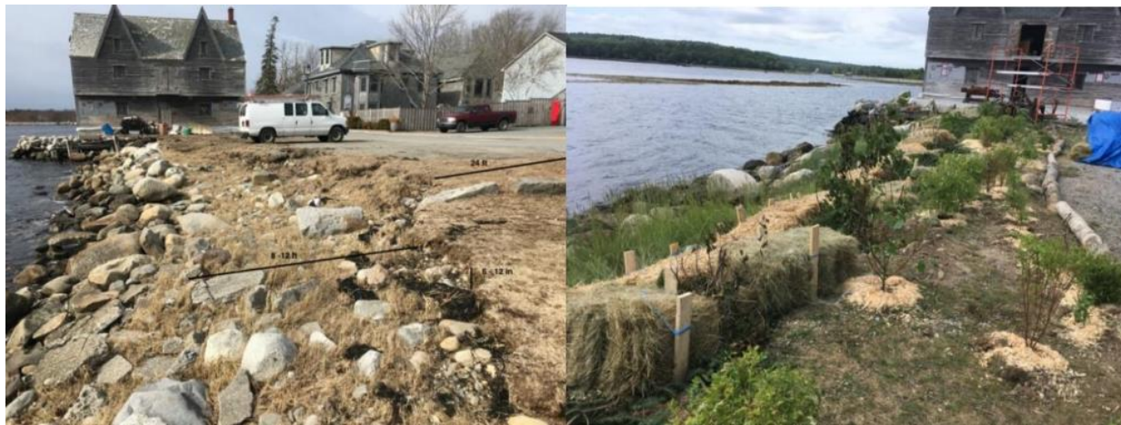
Figure 3.32 Before (March 2020) and after (August 2020) implementation of living shoreline practices to stabilize the bank (Coastal Action, CBWES)
