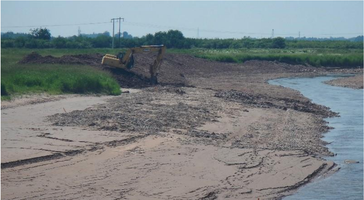
Figure 3.22 Example of a dredging project from a small-scale channel mechanical excavation in Salmon River, NS (Graeme Matheson, Saint Mary's University)
