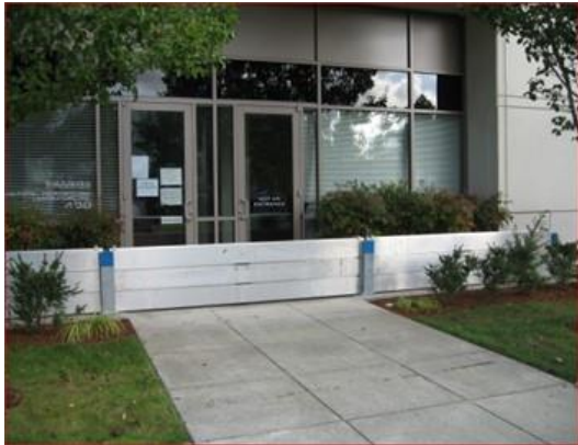
Figure 3.45 Example of a removable floodwall/gate in Maine 48
