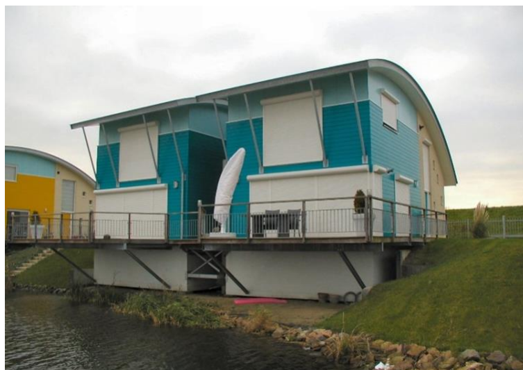
Figure 3.27 Home on an amphibious foundation in Holland (Dura Vermeer)
