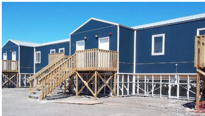
Figure 3.26 A multipoint foundation spreading the weight of a building over a wide area, allowing the structure to be more adaptable (Triodetic Multipoint Foundations) 30
