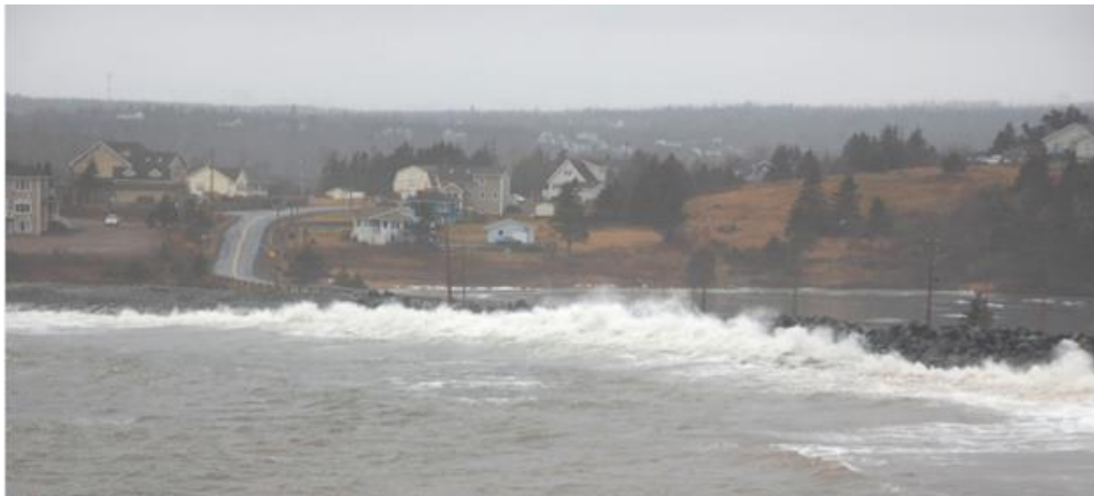
Figure 3.36 Cow Bay Causeway experiencing a storm in 2010.
