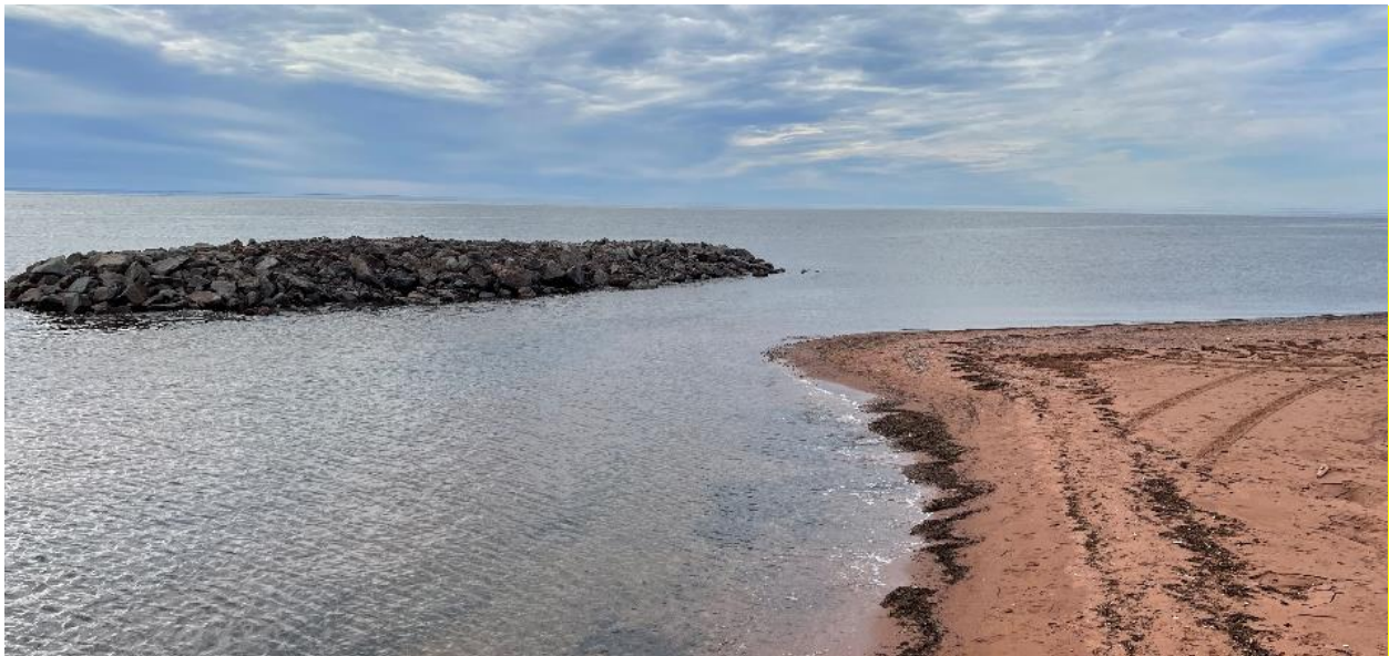
Figure 3.16 Breakwater constructed to mitigate erosion at West Point, PEI (Vincent Leys, CBCL Limited)
