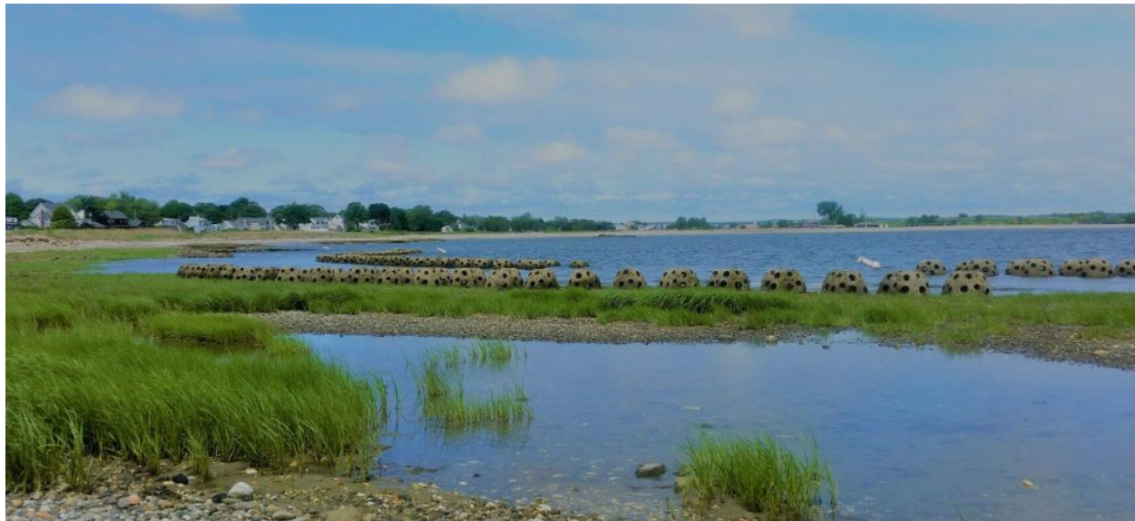
Figure 3.38 Concrete reef ball installation along Stratford Point (National Audubon Society Inc., 2020)
