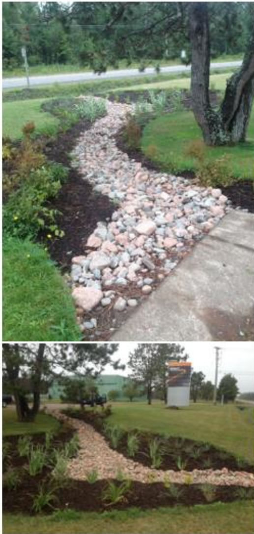
Figure 3.50 Bio-infiltration zone installation at Debert Industrial Park, Debert, NS (Tracey MacKenzie, 2015)
