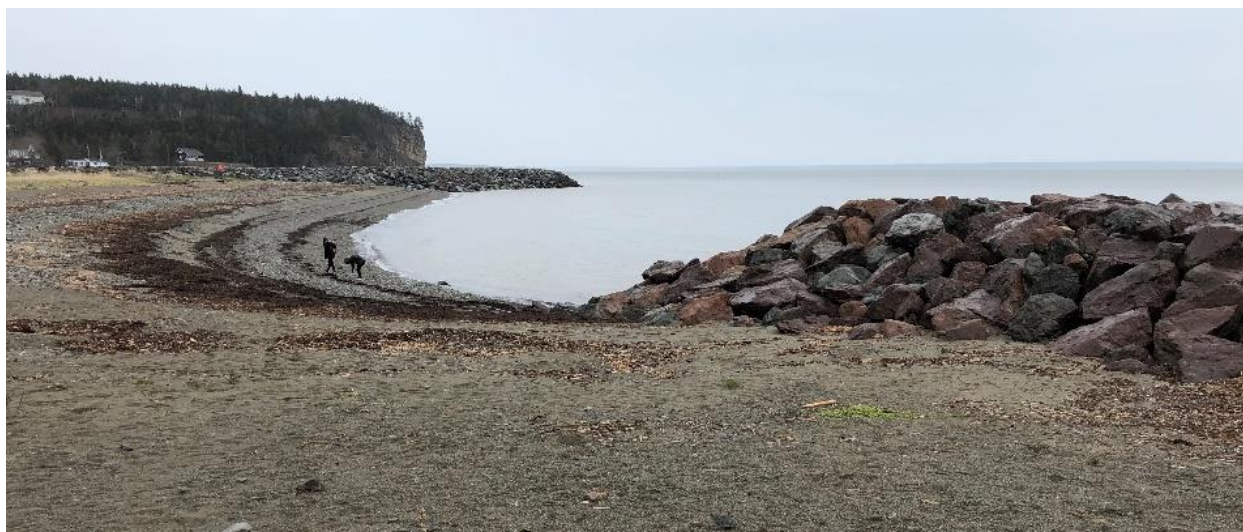
Figure 3.33 Brise-lames au parc national Fundy (Vincent Leys, CBCL Limited)
