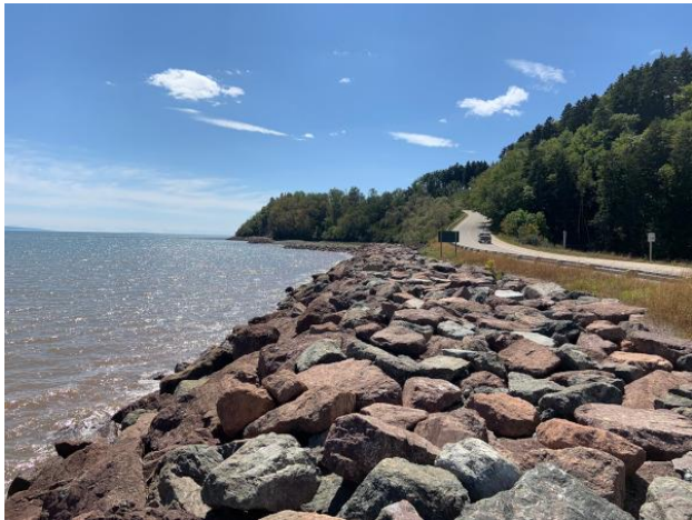
FIGURE 2. SHORE PARALLEL ENGINEERED STRUCTURES (REVTMENTS, SEAWALLS, NEARSHORE BREAKWATER). IMAGE SOURCE CLIMATLANTIC COASTAL ADAPTATION TOOL (2023)
